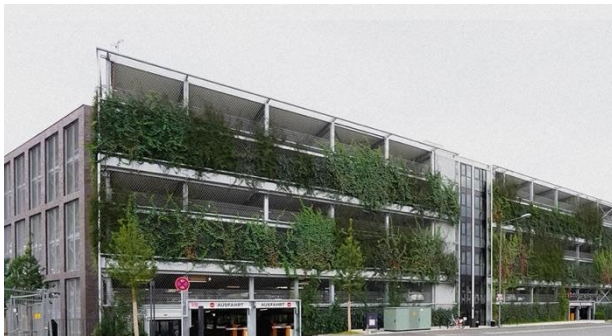
Figure 10 Green façade at a parking garage in Köln Mühlheim
